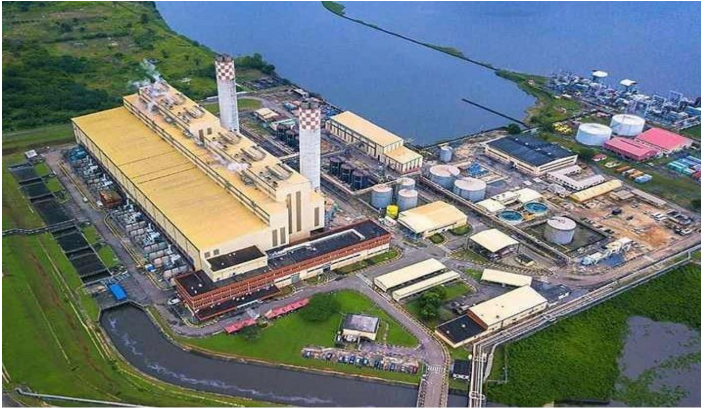
Figure 8. Egbin power plant. Image source: https://www.sahara-group.com/
