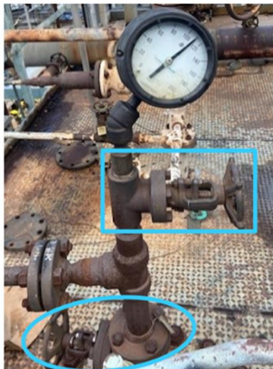
Figure 1. Valves isolating the pressure gauge
